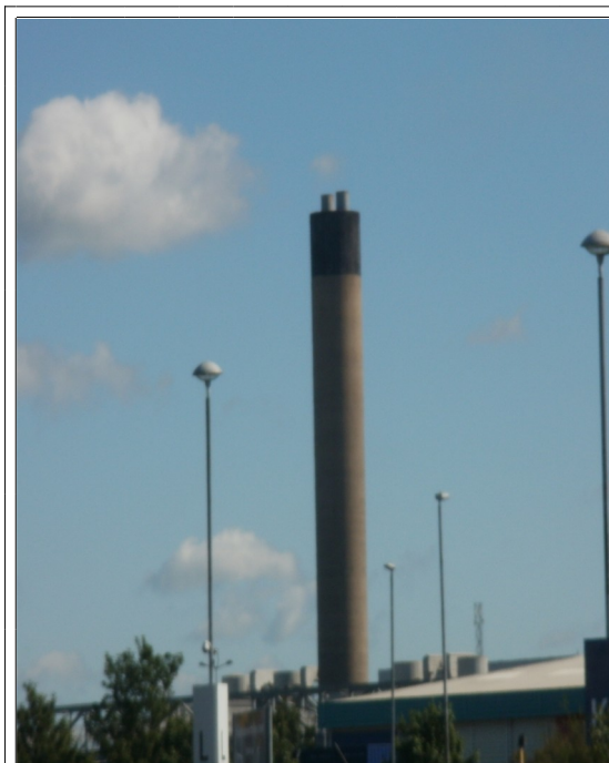
The Edmonton stack is due for demolition in 2020 but will the replacement stack be located in Friern Barnet?
