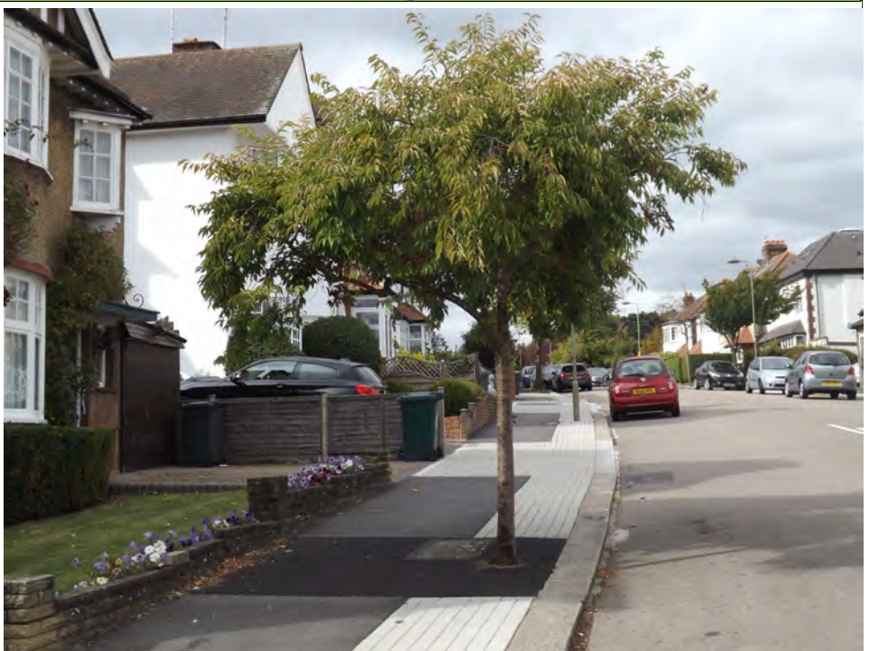
The darker surface around the tree shows the use of the new, porous Micro Surfacing
